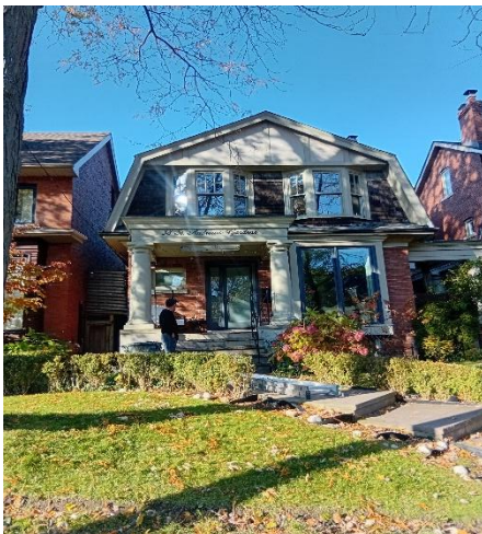
Front, facing North.
