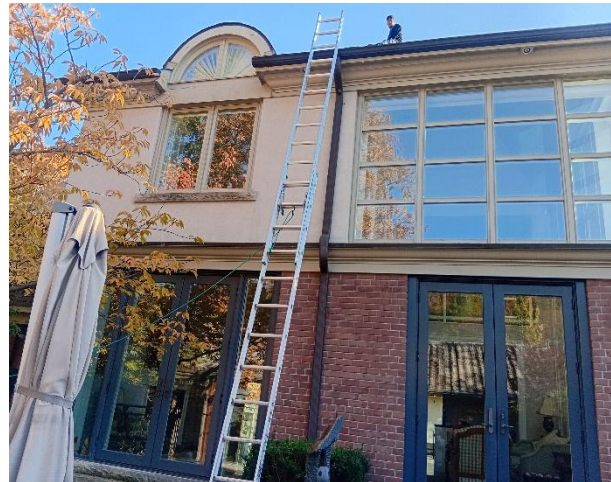
Rear, facing South.
